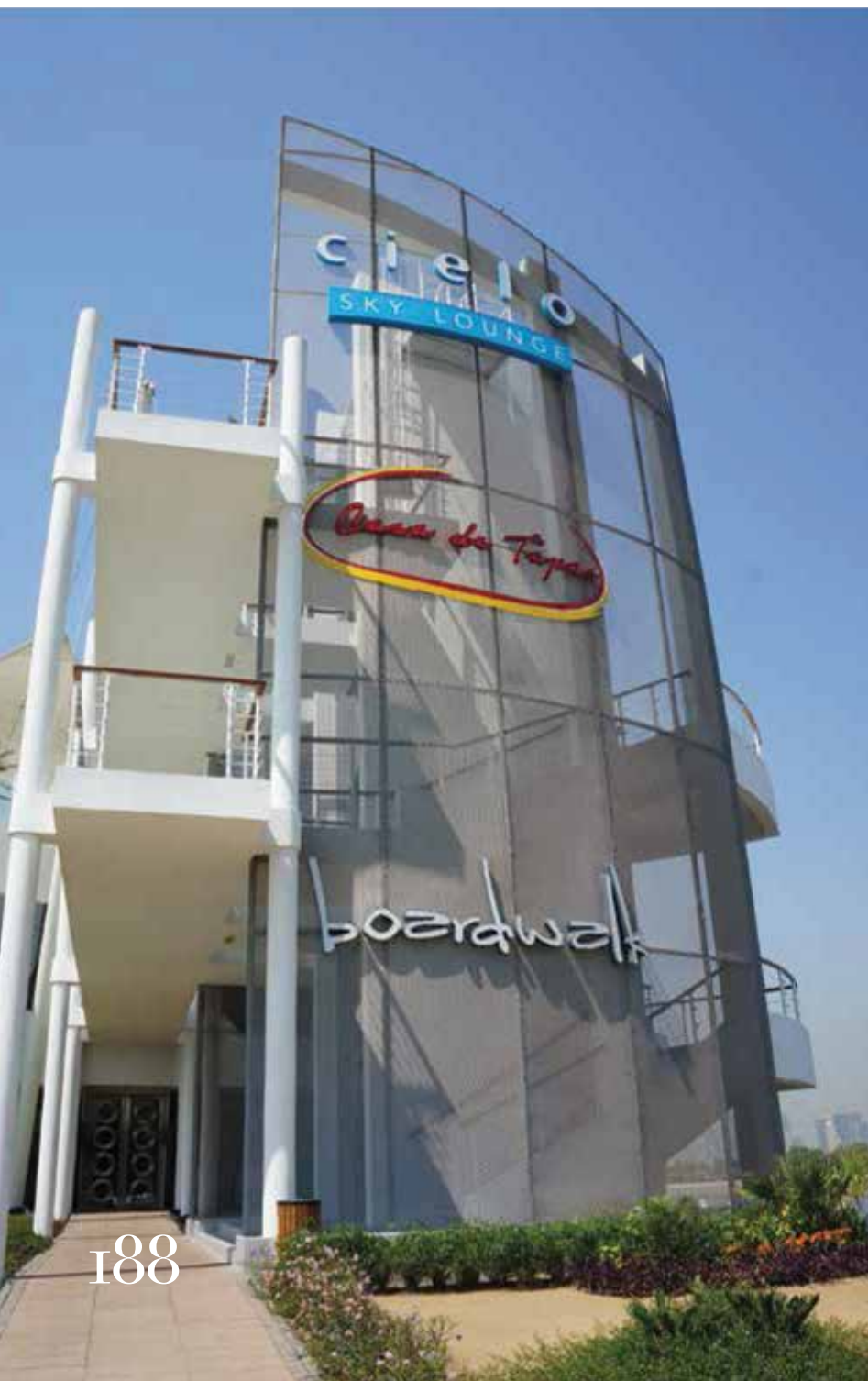
DUBAI CREEK - FACADE CLADDING VIEW - UAE
